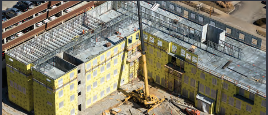
Hambro D500 composite floor system on load-bearing steel stud walls
