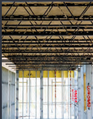
Hambro D500 composite floor system on load-bearing steel stud walls
